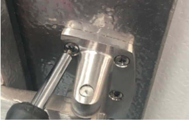
1. Re-tightening latches, strikes etc.
