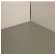
Floor with PVC coating
