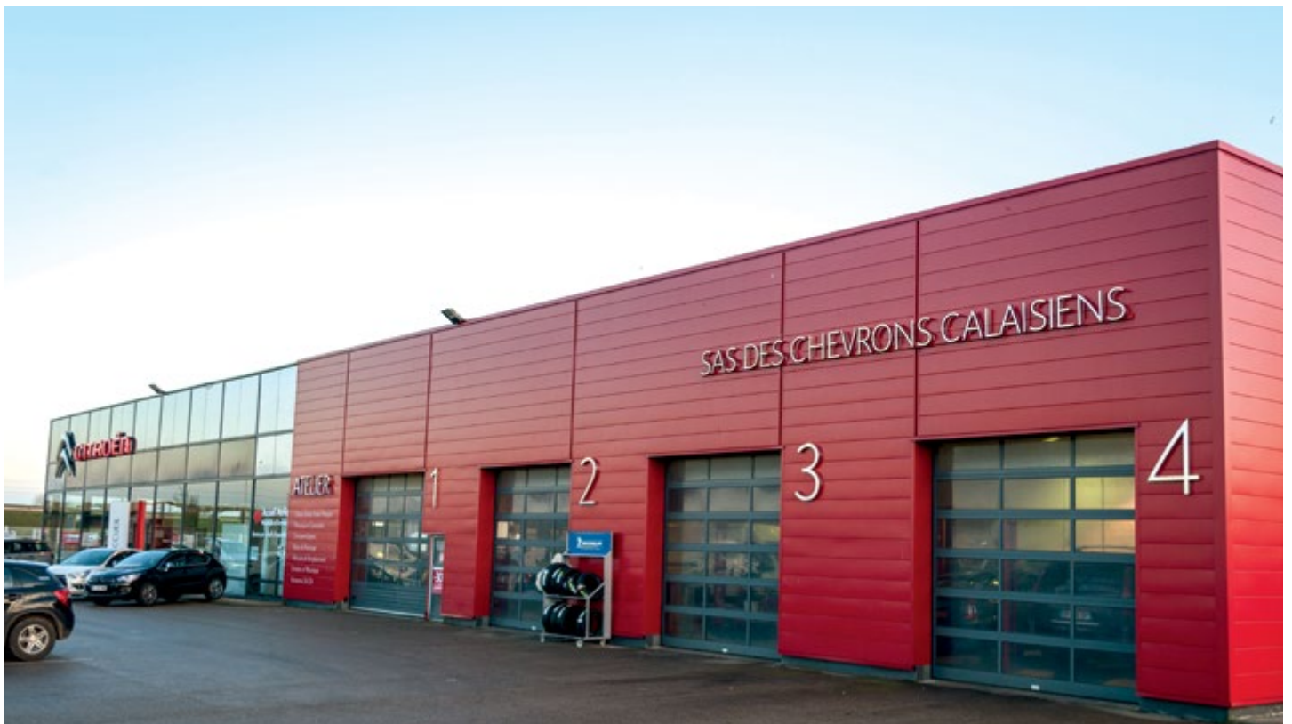
Images courtesy of Architect: Toth-Wallyn
